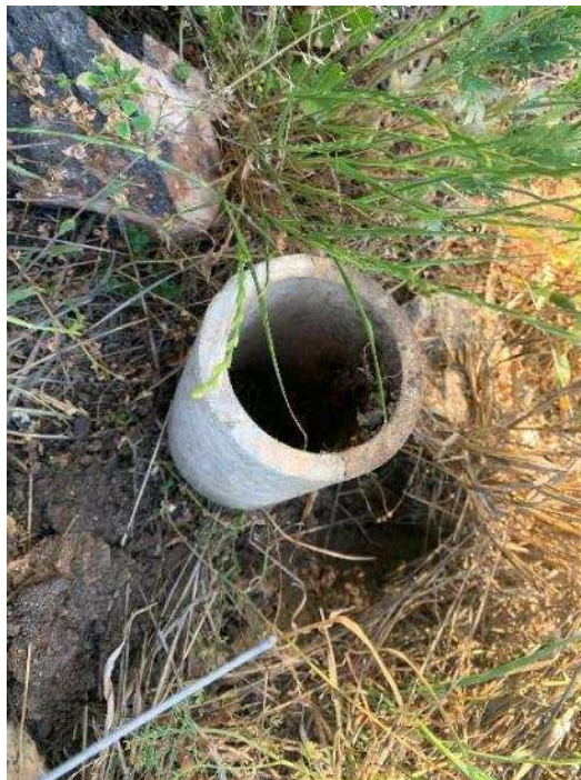
Image 7.3.2.2 View of potential ACM pipe at ACM01 location
