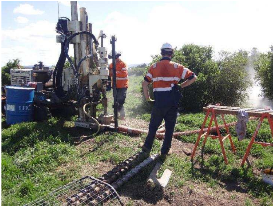
Image 7.6.1.3 View of second round of drilling at MW04 (image shows air hammering being conducted).
